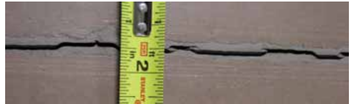
Adhesive joint filler separation (joint wall)
