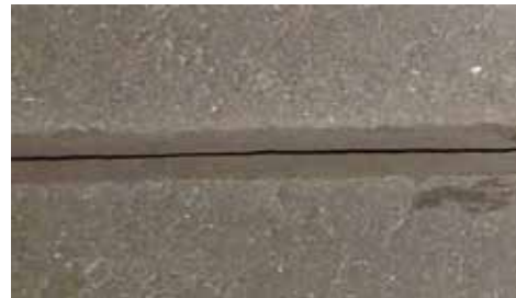
Cohesive joint filler separation (internal)
